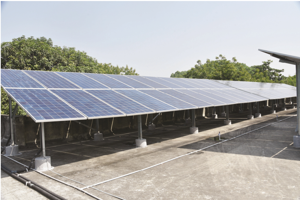
Installation Solar panels for the capacity of 1.434 MW
