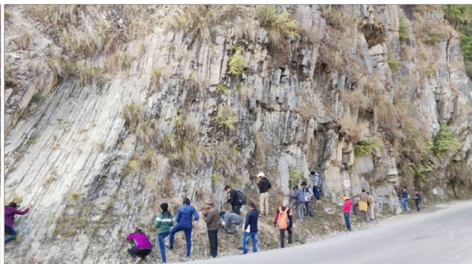
Students identifying the mode of failure with detailed engineering geological mapping at Munsiyari, Uttarakhand
