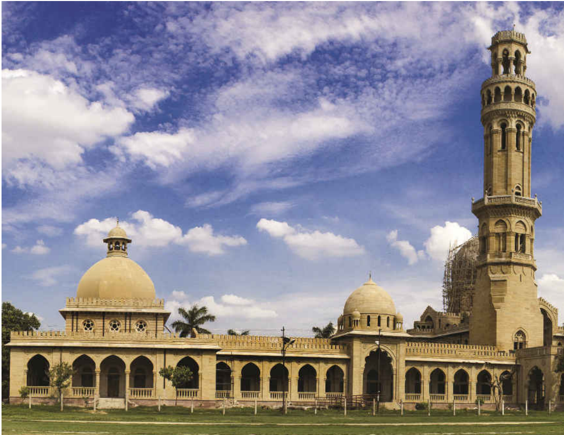
Renovated Vijayanagaram Hall
