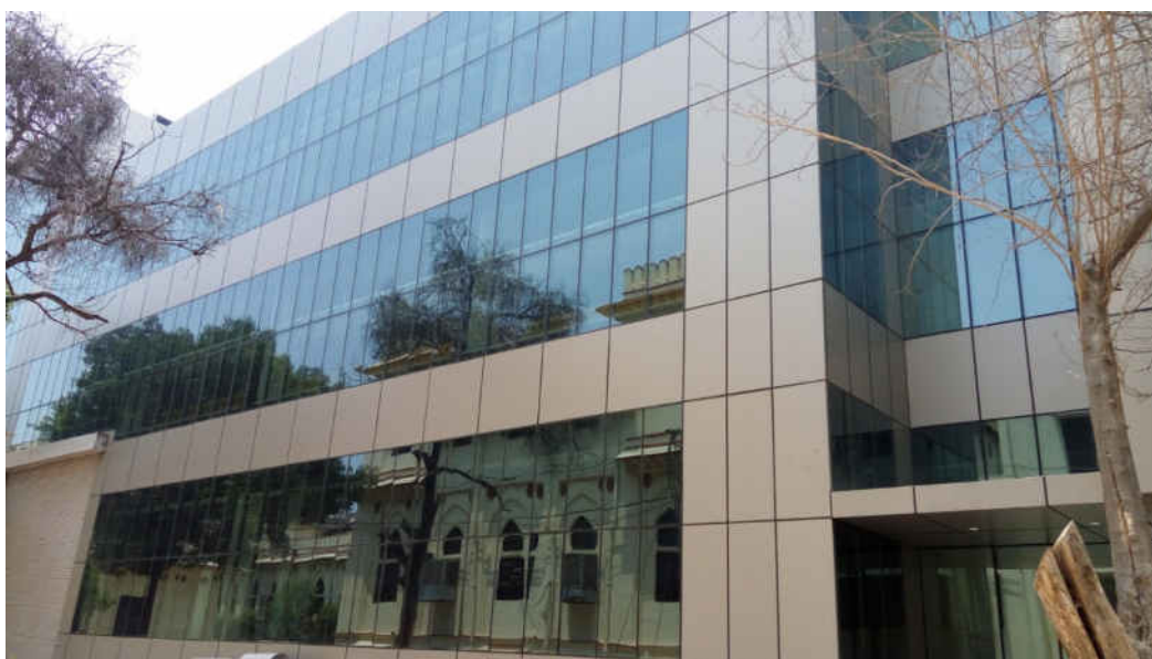
Building for Accelerator Center (Start date for construction 10.04.2014- Completion August 2015) by RITES INDIA
